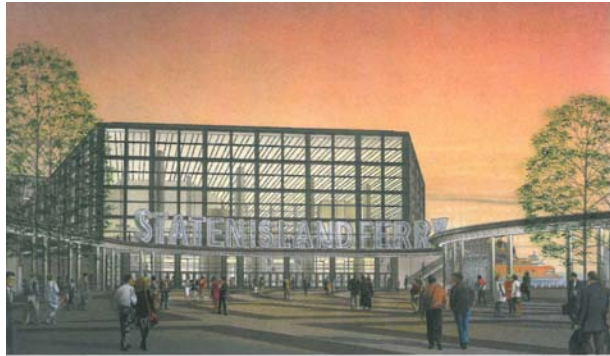
The terminal's coated-glass walls (left and below left) are energy efficient and provide astonishing views of the city and harbor surrounding its prime location (bottom). Rooftop photovoltaic cells (below) generate enough energy to light the building's offices.
